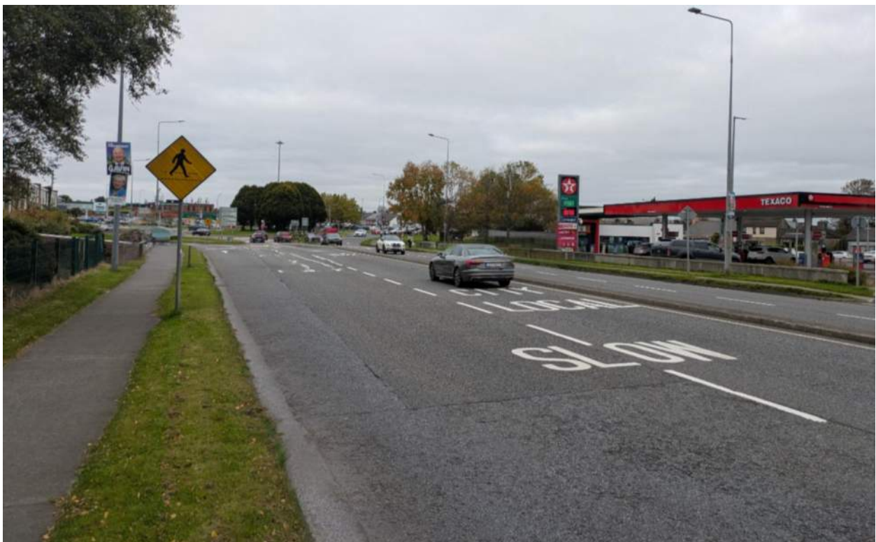
Figure 3-4: Dublin Road approach to Parkway Roundabout looking West
