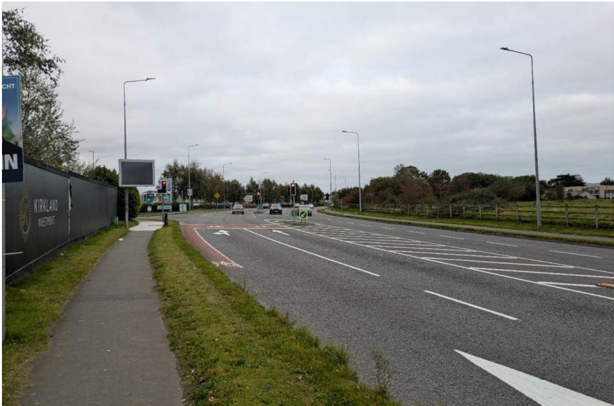
Figure 3-3: Dublin Road approach to Signalised Junction looking West
